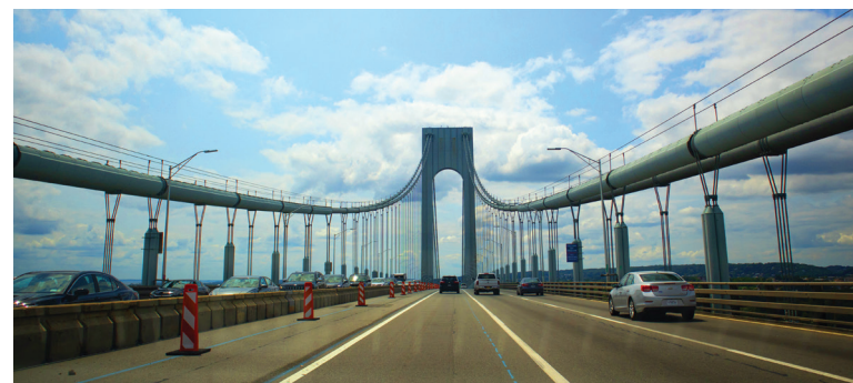
View of the Verrazzano-Narrows Bridge
