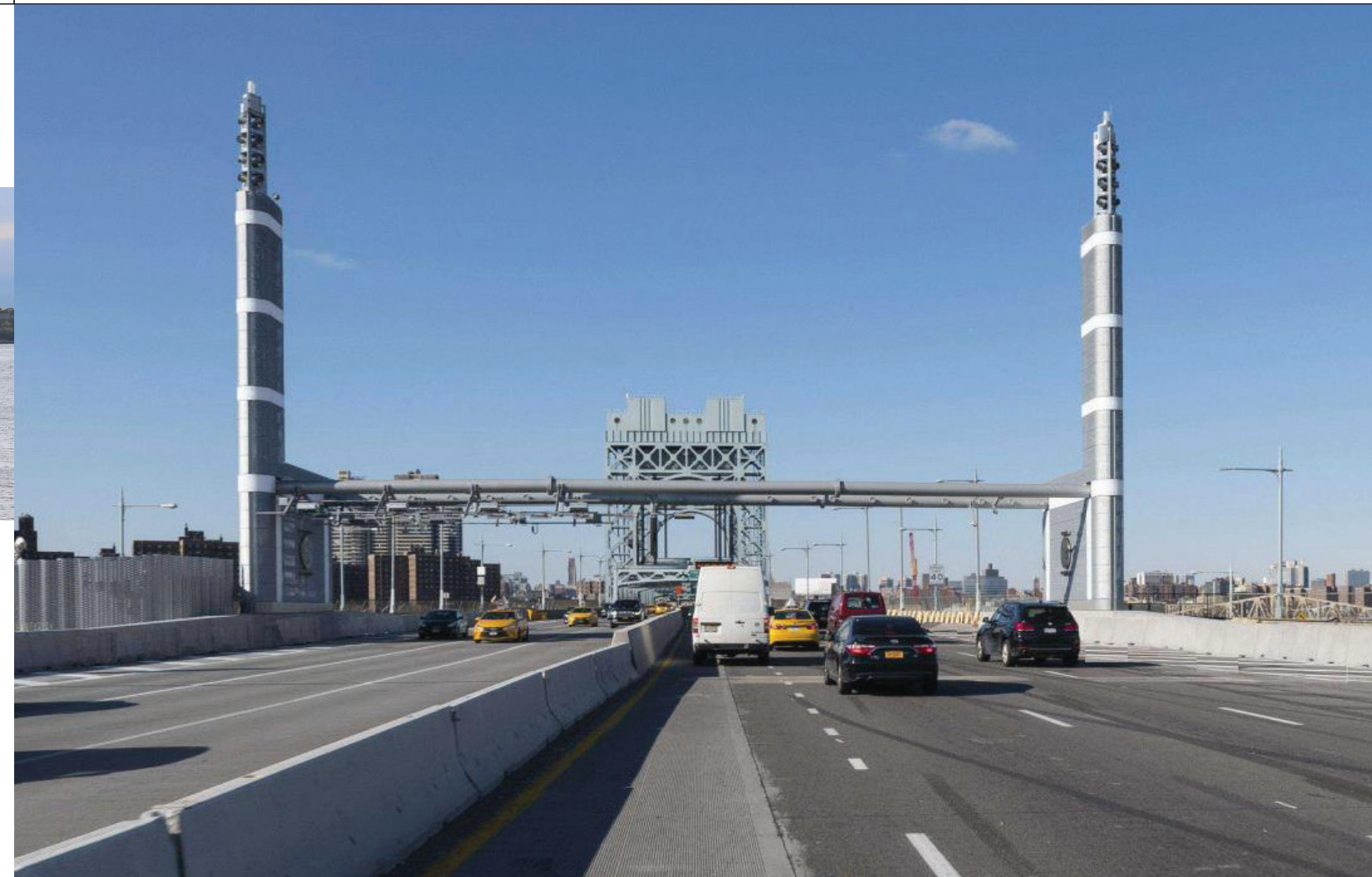
Cashless tolling and Gateway Towers at the Robert F. Kennedy Bridge
