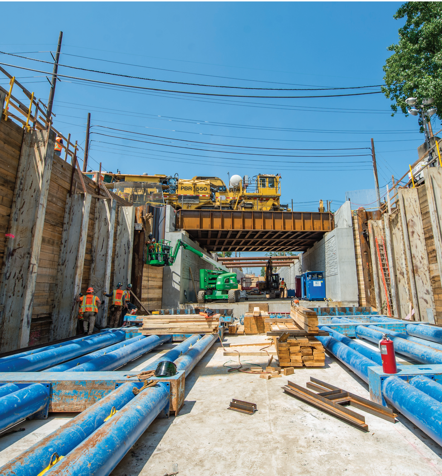
Above, LIRR Third Track Construction Photo
