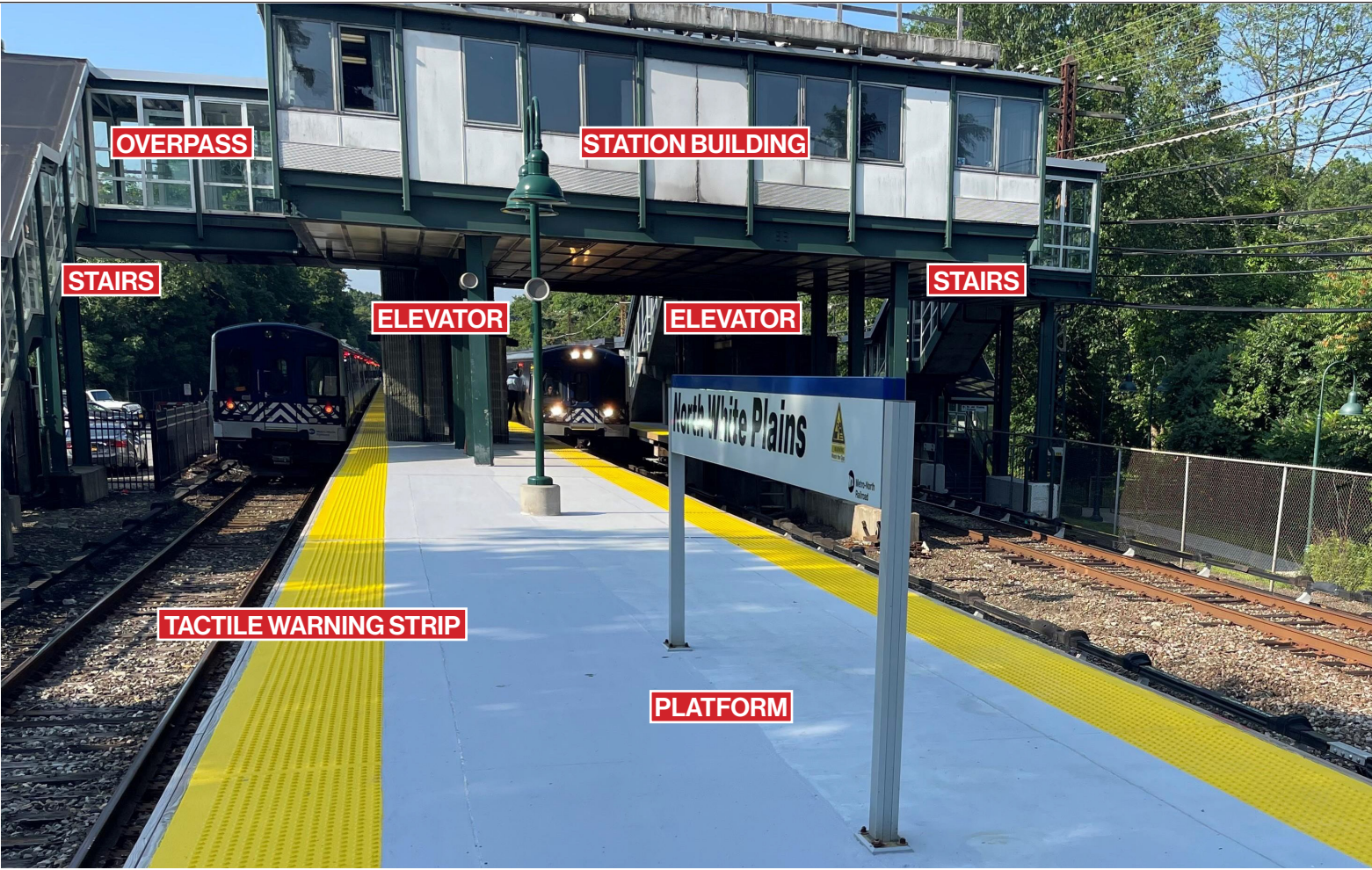
North White Plains Station with station components
