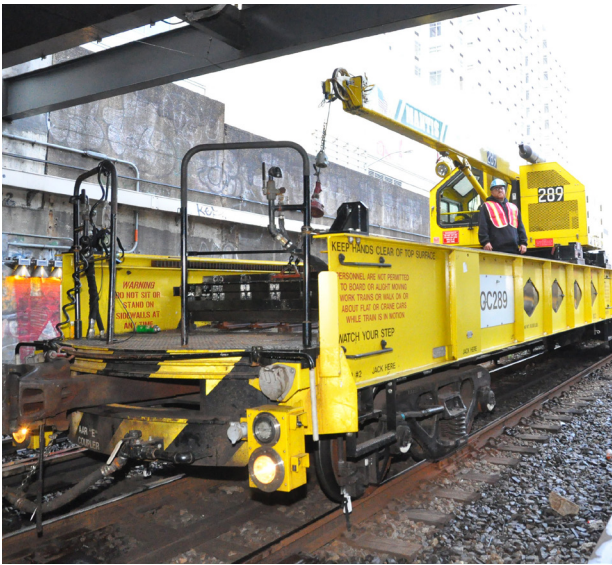
Work train with crane
