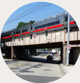
Undergrade bridges Allow an obstacle to pass under the railroad (i.e., the tracks are on the bridge structure).
