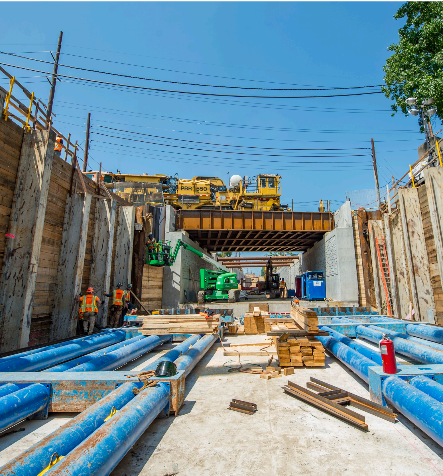
Above, LIRR Third Track Construction Photo
