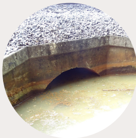
Culverts Are designed to allow water to flow underneath tracks to manage drainage and prevent flooding.
