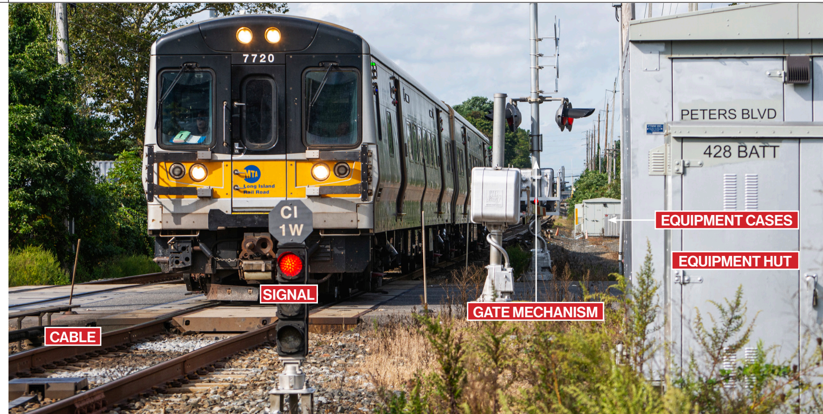
Above, standard LIRR signals system annotated with signals components
