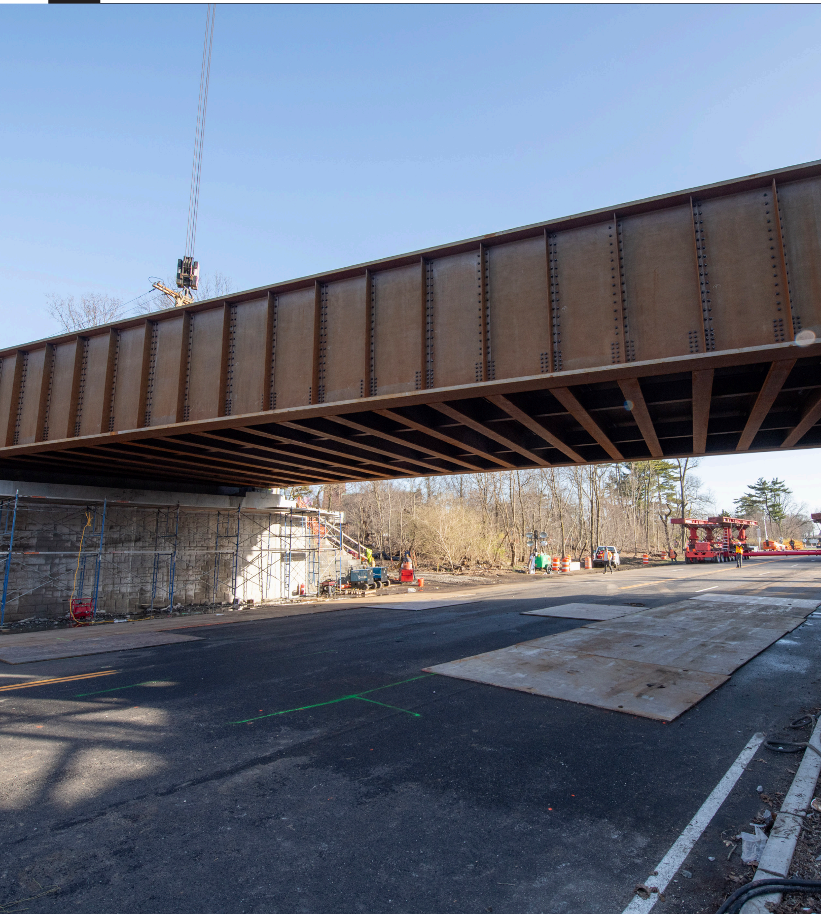
Cherry Valley Avenue Bridge
