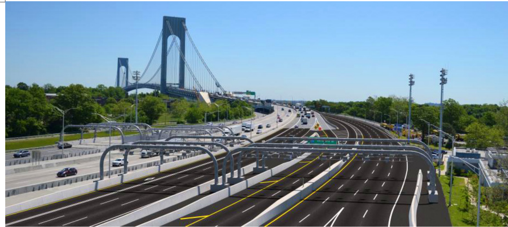
Split tolling at the Verrazzano-Narrows Bridge
