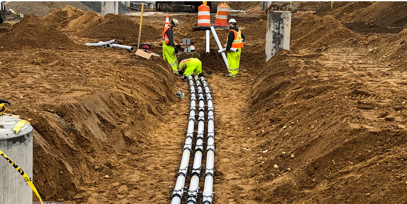
Below, installation of communications ductwork
