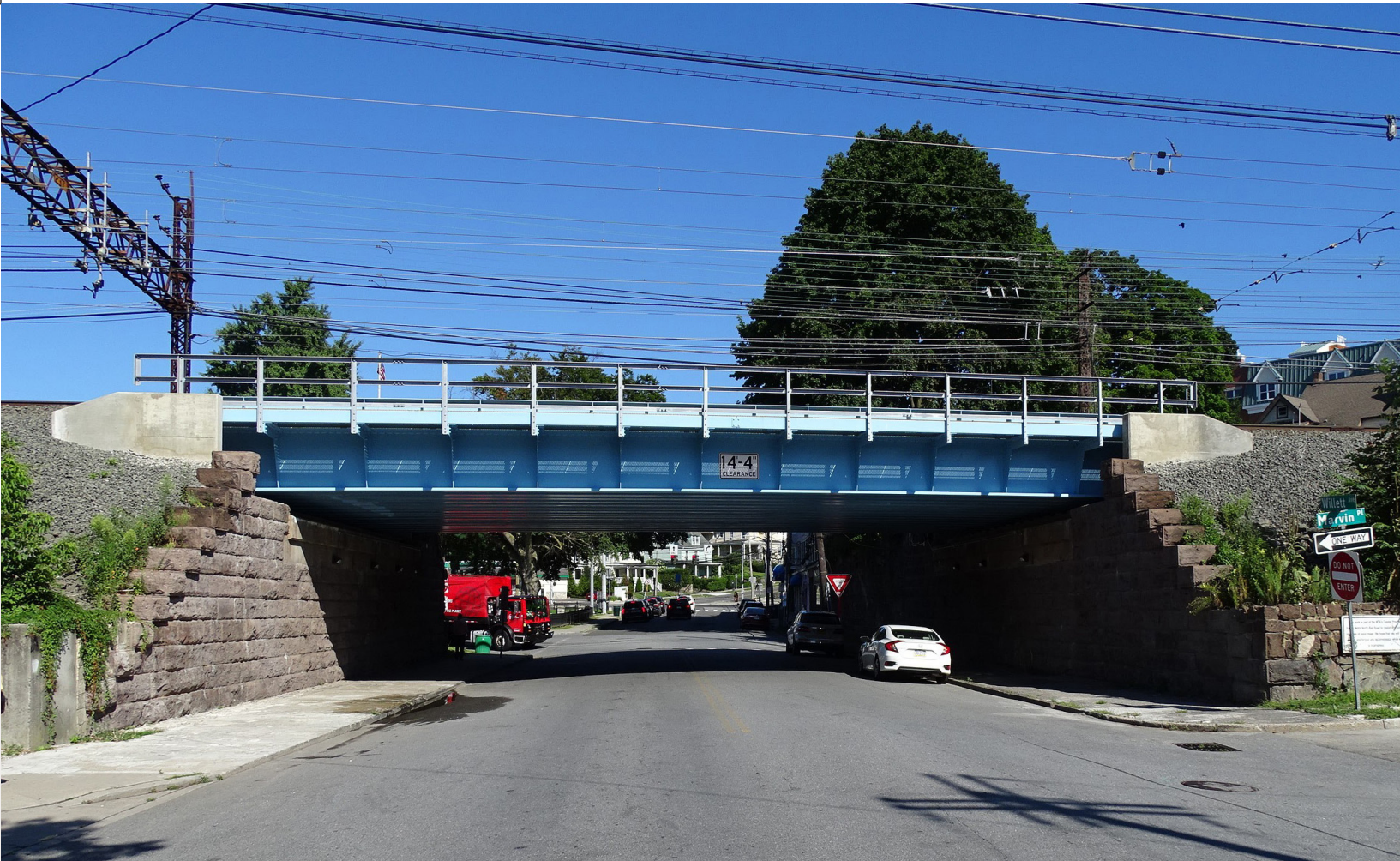
Willet Ave undergrade bridge
