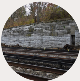
Retaining walls Built to hold back soil and provide support for our elevated structures.
