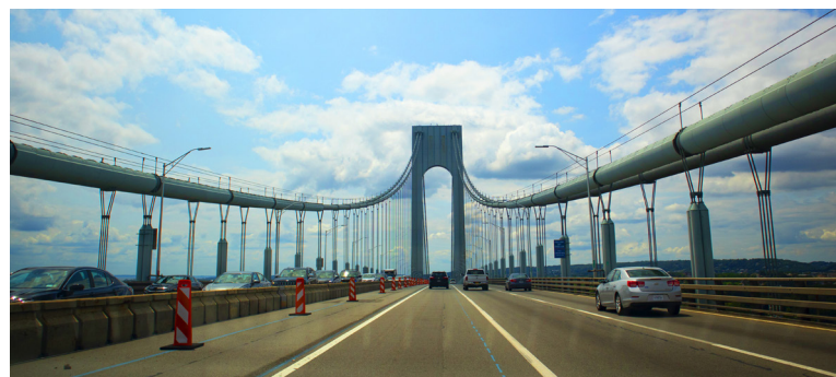
View of the Verrazzano-Narrows Bridge
