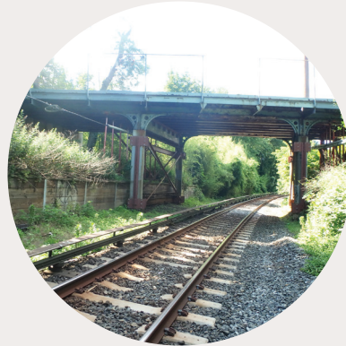
Overgrade bridges Allow the obstacle to pass over the railroad (i.e., the roadway is on the bridge structure).
