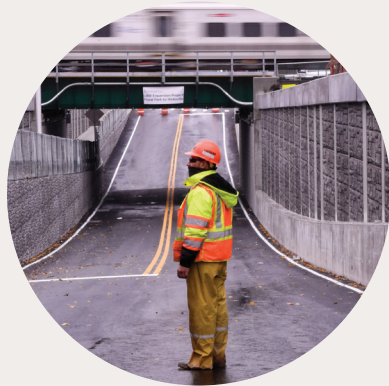
Undergrade bridges Allow an obstacle to pass under the railroad (i.e., the track(s) are on the bridge structure).
