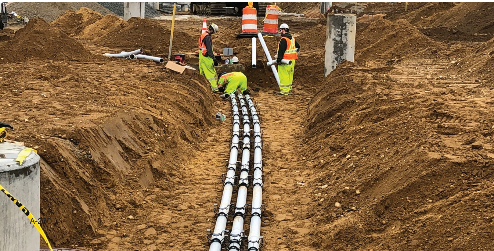
Below, installation of communications ductwork
