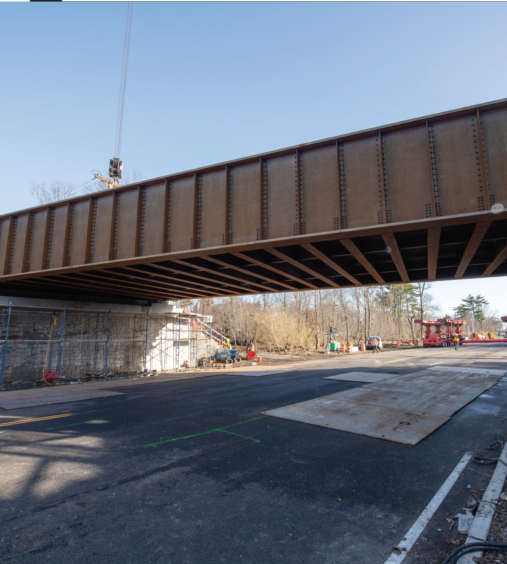
Cherry Valley Avenue Bridge
