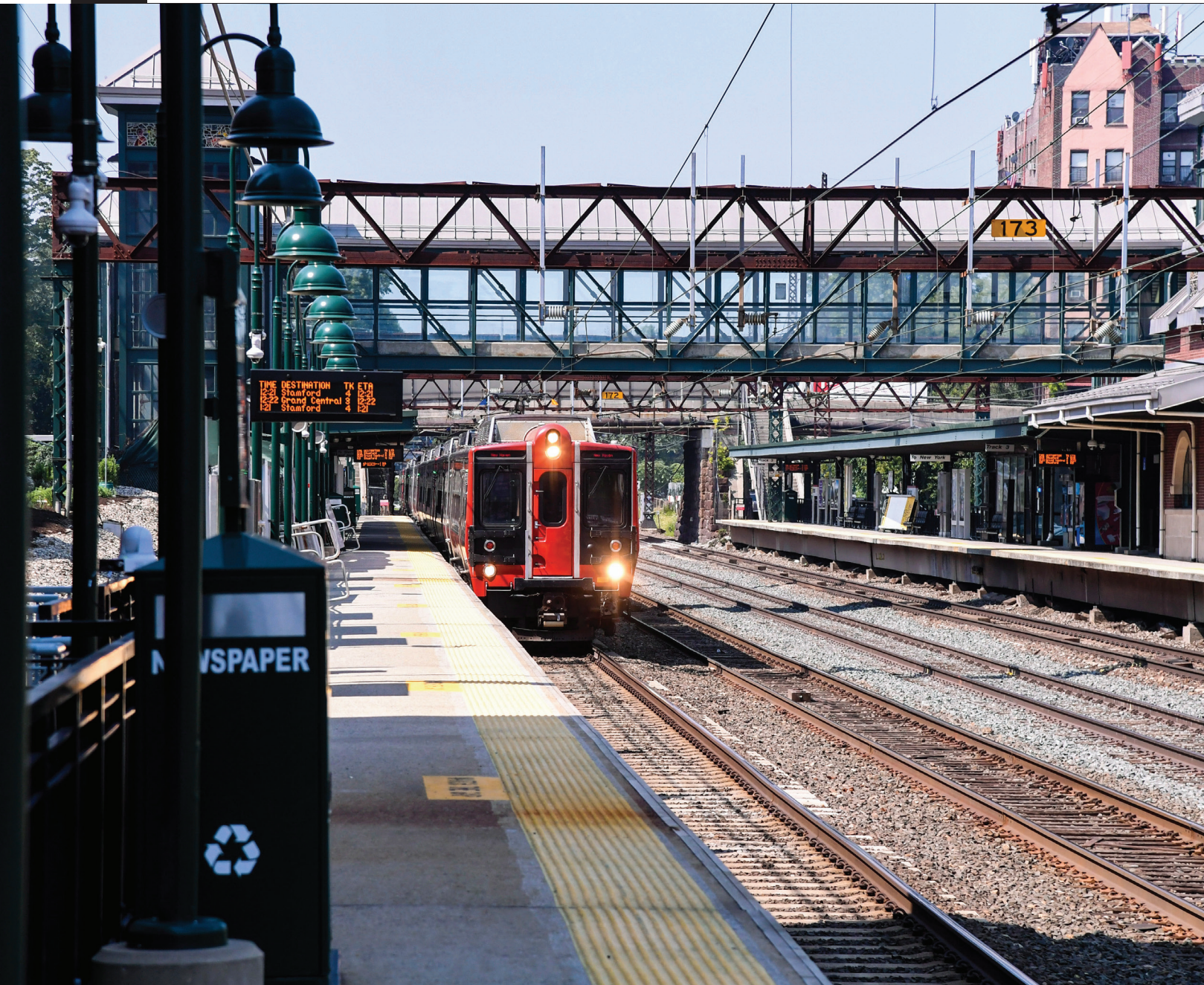
Harrison Station on the New Haven Line
