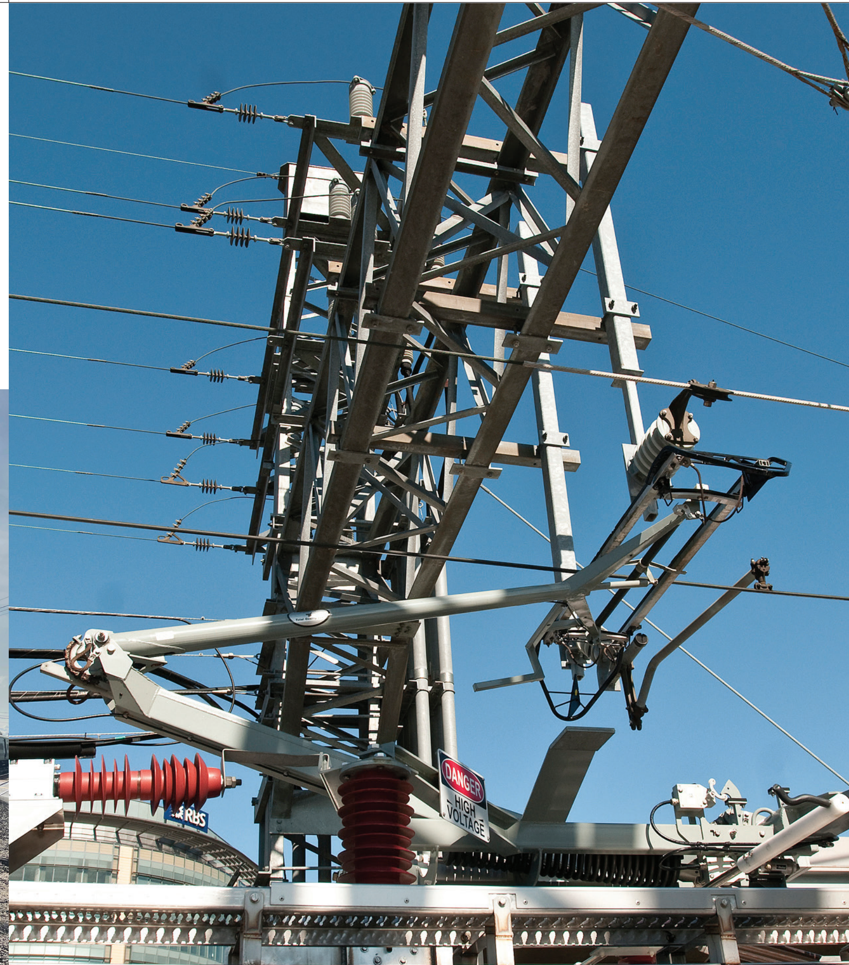
Overhead catenary power system, New Haven Line
