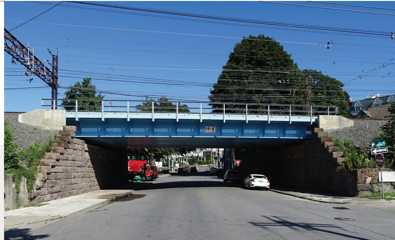
Willet Ave undergrade bridge
