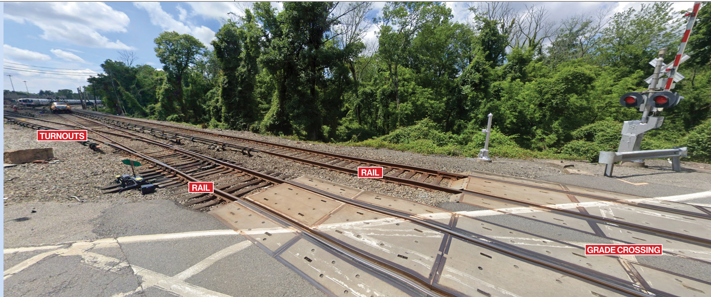
Harlem Line intersection with Virginia Road (White Plains), Source: Google Streetview
