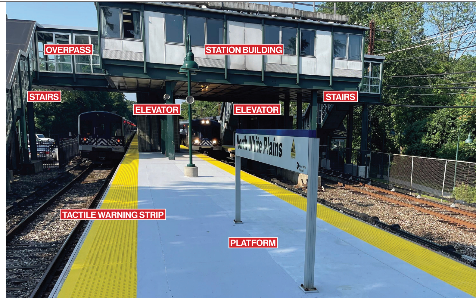
North White Plains Station with station components
