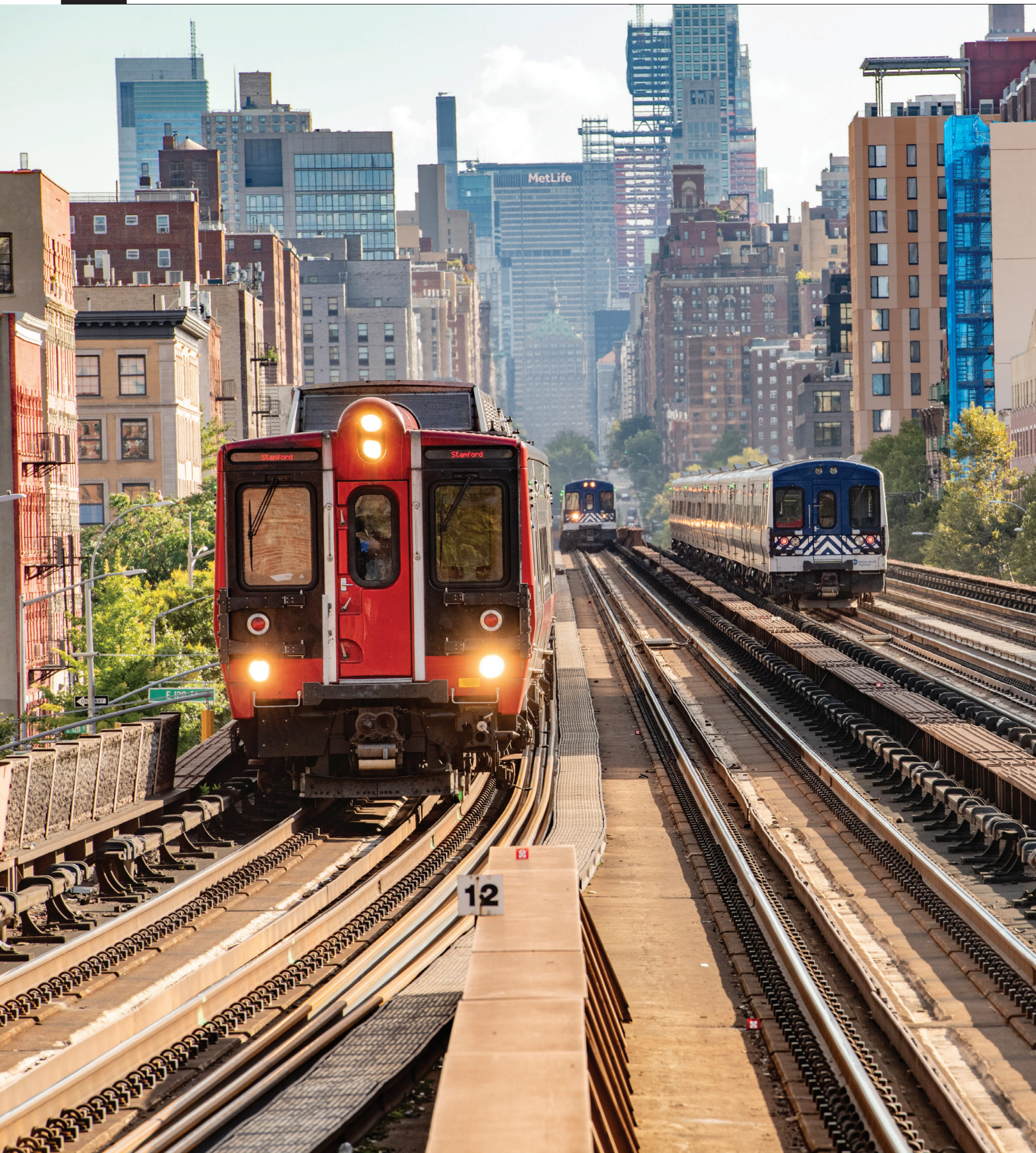
EMU trains on the Park Avenue Viaduct
