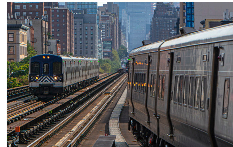
Metro-North trains on the viaduct north of Grand Central Terminal
