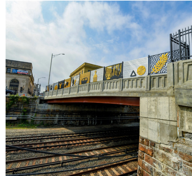
Metro-North overhead rehabilitation
