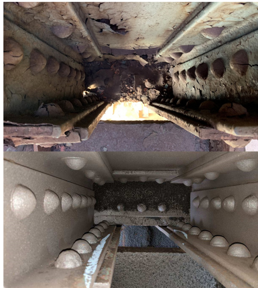
Before and after photos of aged paint removed using abrasive blasting
