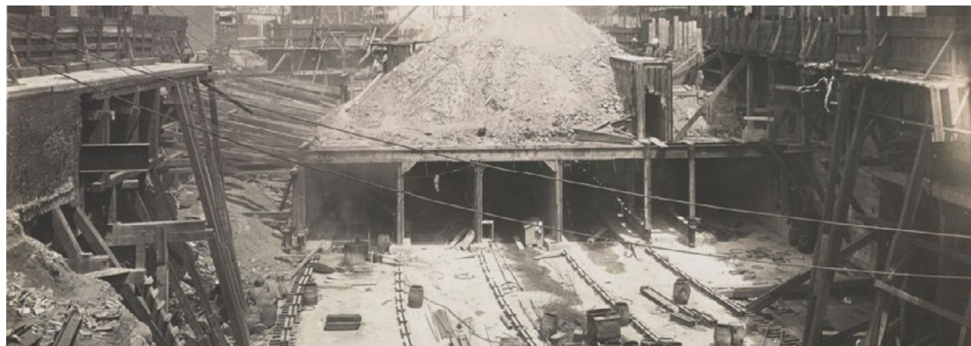
DeKalb Interlocking under construction in 1911
